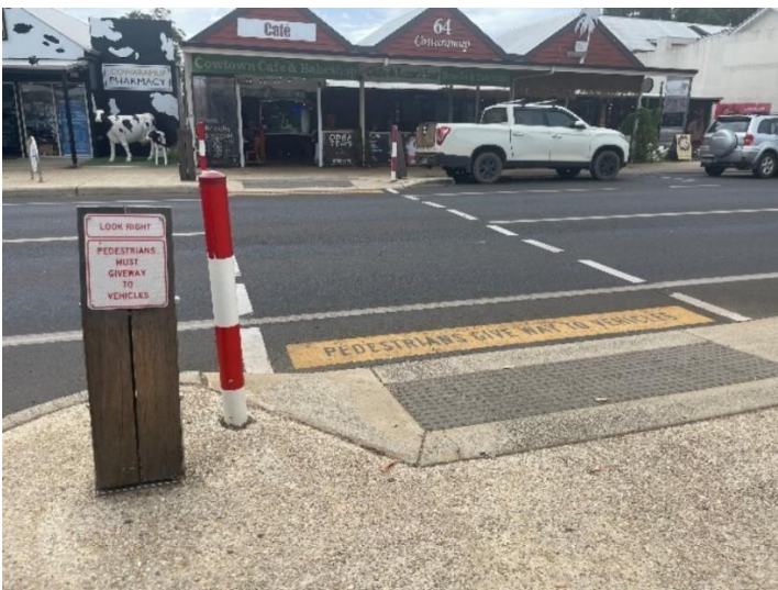
Figure 2-19 Pedestrians Give Way to Vehicles
