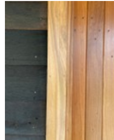
New & old timber
