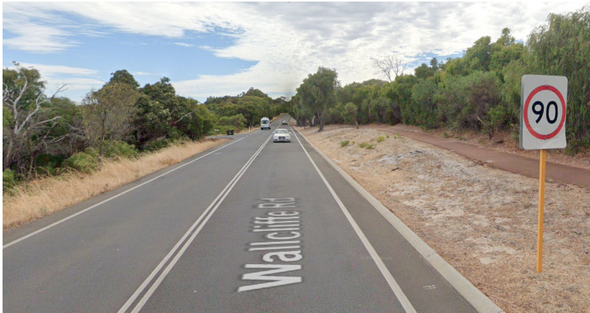
Figure 4: Wallcliffe Rd (looking northeast to existing driveway)
