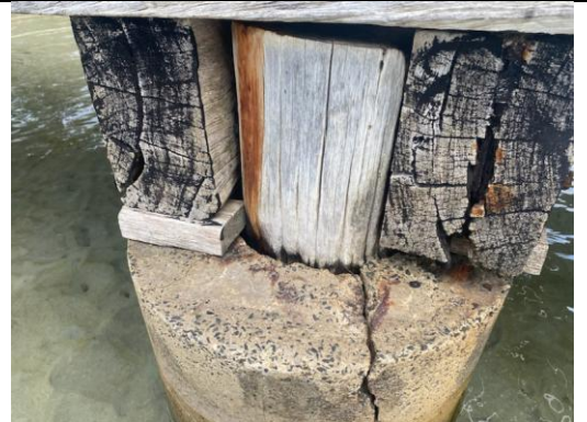
P12 Headstock – ends severely split
