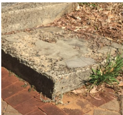
Transition from stairs to paved area (public toilet access)
