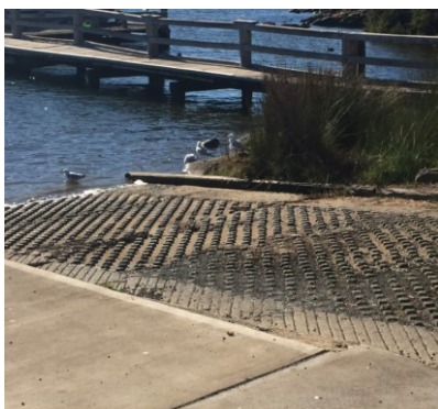
Boat ramp – water access
