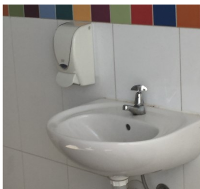
Sink and tiling within public toilets
