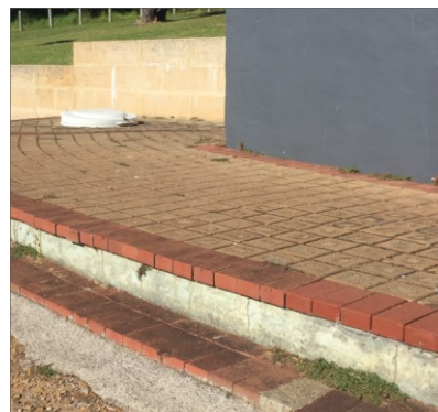
Public toilet access from roadway
