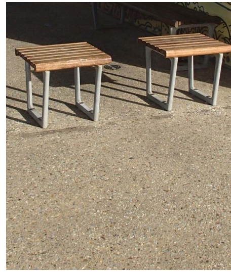
EXISTING EXPOSED AGGREGATE CONCRETE
