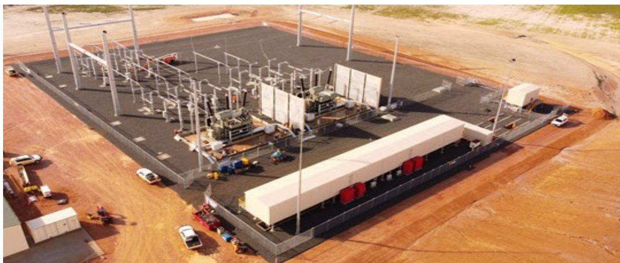
Figure 8 Typical Substation Layout
