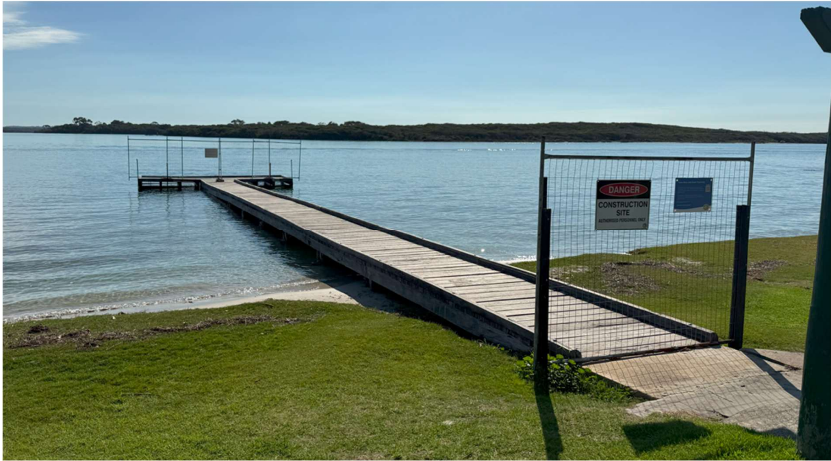
Figure 2.1 Turner Street Jetty (May 2025)
