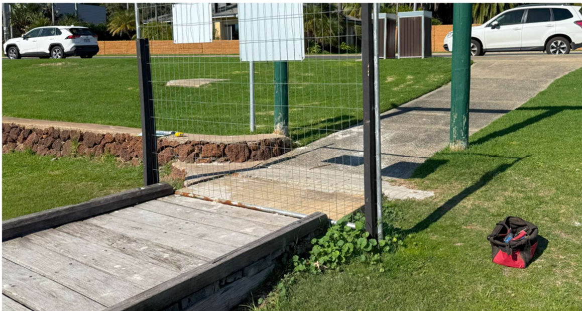
Figure 2.4 Jetty Abutment & Land Approach
